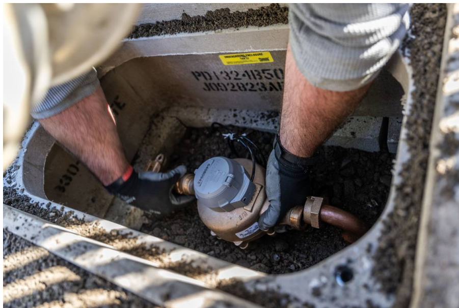
Mathew Harrington, who works for the City of Sacramento Department of Utilities, installs a water meter earlier this month at one of the last city homes without one. Hector Amezcua hamezcua@sacbee.com
