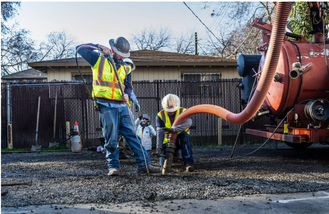
Mathew Harrington, who works for the City of Sacramento Department of Utilities, installs a water meter earlier this month at one of the last city homes without one. Hector Amezcua hamezcua@sacbee.com
