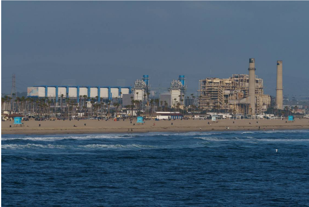
The AES Huntington Beach Energy Center, shown in May, was the proposed site of the Poseidon Huntington Beach Seawater Desalination Plant. The California Coastal Commission rejected the proposal a few days later. Damian Dovarganes AP
