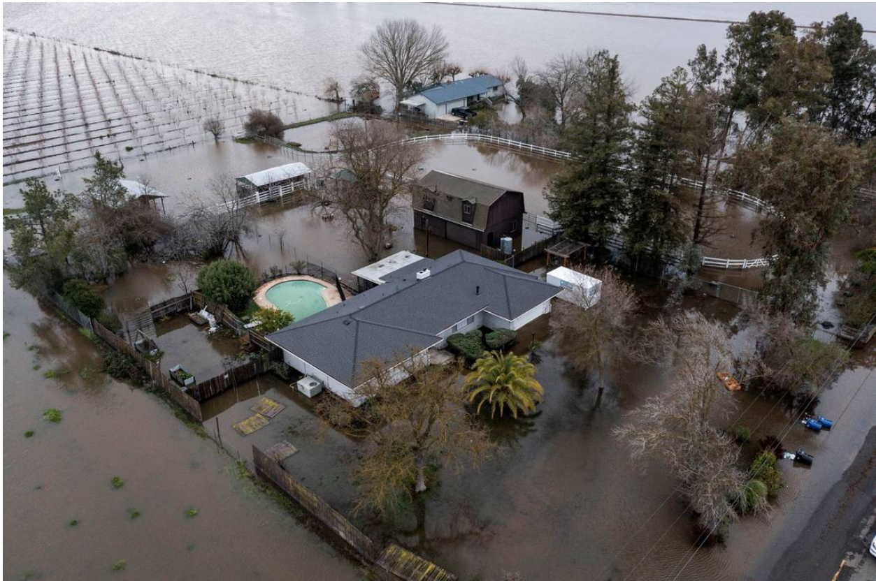
An aerial view shows a flooded home in Point Pleasant on Jan. 2 after record-setting rainfalls caused levee breaks at the Cosumnes River. Hector Amezcua hamezcua@sacbee.com
