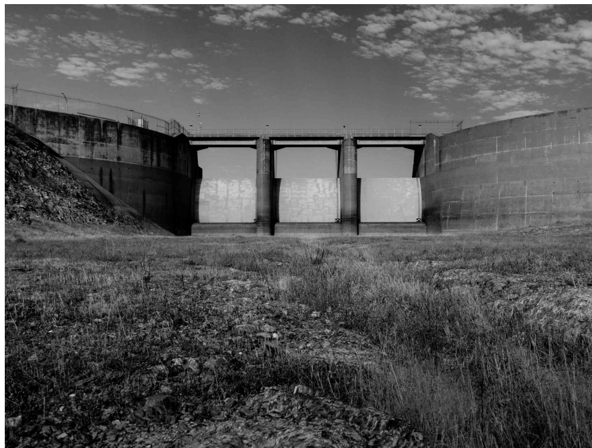
The New Don Pedro Dam spillway.
