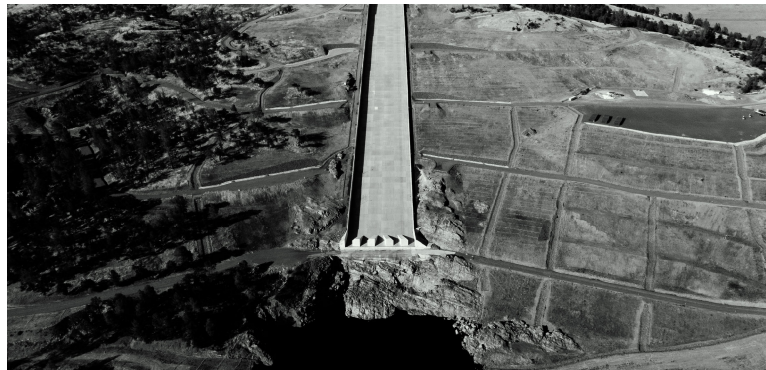
[Reconstructed Oroville Dam main service spillway]
