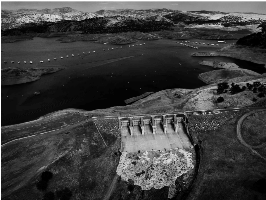
The spillway of the New Exchequer Dam.
