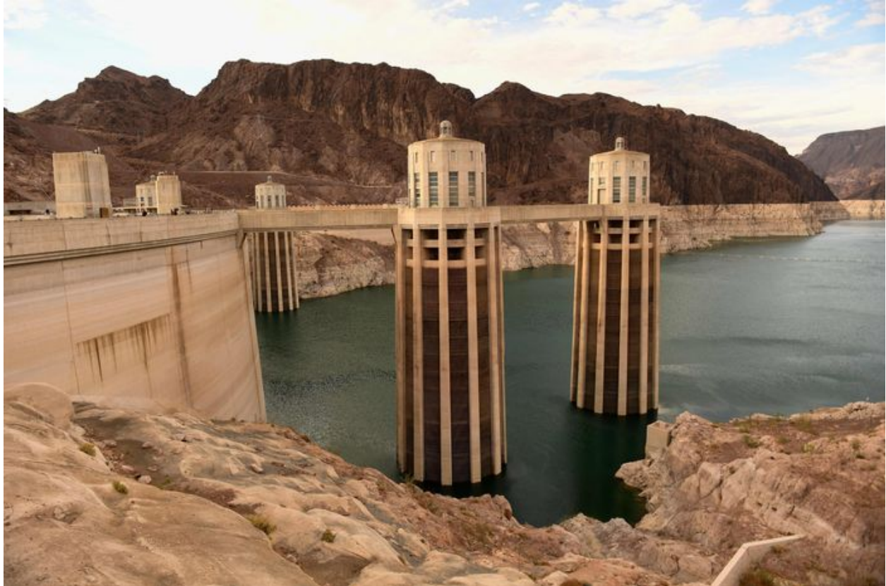
Intake towers at the Hoover Dam at the Nevada-Arizona state border.
