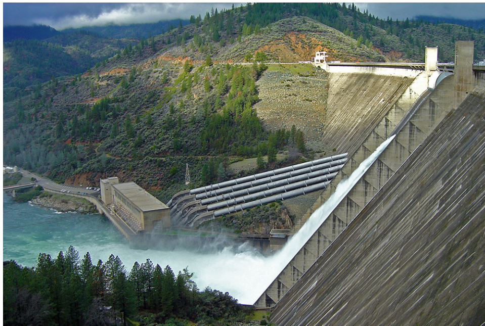
Shasta Dam, California
