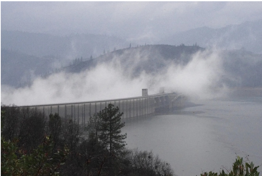
Federal officials want to raise the height of Shasta Dam to store more water in Lake Shasta. Damon Arthur, Record Searchlight
