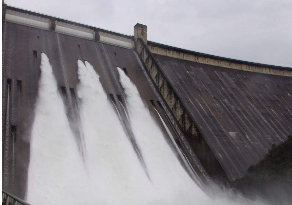
Ports on the Shasta Dam spillway send thousands of gallons of water down the face of the dam Monday. The amount of water released rose to 30,000 cubic-feet per second. Damon Arthur/Record Searchlight
