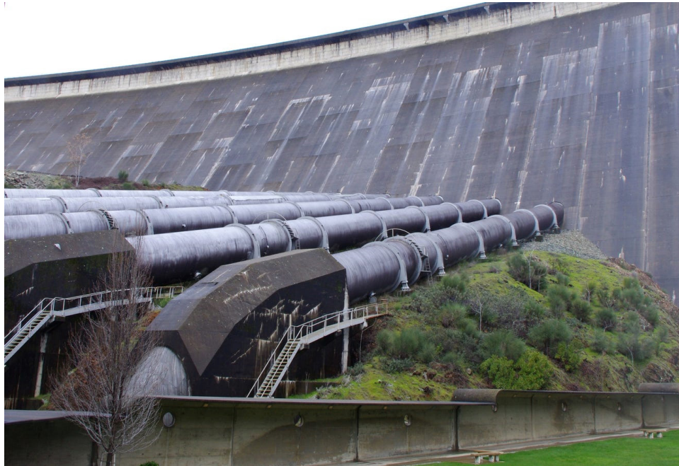
In addition to increasing the amount of water coming down the spillway of Shasta Dam, four of the five turbines were generating electricity Tuesday. Damon Arthur/Record Searchlight
