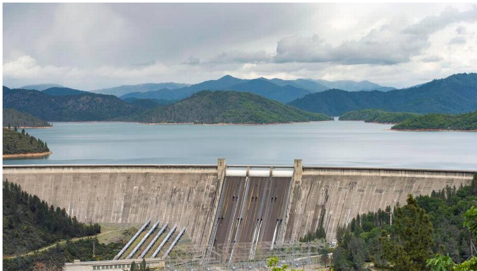
Republicans in Congress authorized spending $20 million to study raising Shasta Dam by 18.5 feet. If ever fully approved, the $1.3 billion project would flood a stretch of the McCloud River, a wild and scenic river that's sacred for a Native American tribe. Randy Pench Sacramento Bee file
