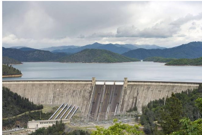
[In 2018] Republicans in Congress authorized spending $20 million to study raising Shasta Dam by 18.5 feet. If ever fully approved, the $1.3 billion project would flood a stretch of the McCloud River, a “wild and scenic river” that’s sacred for a Native American tribe. Monday, April 16, 2018 in Shasta County, Calif
