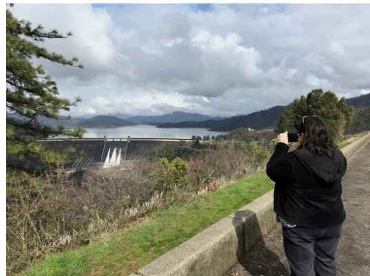
Denise Miraldi of Fairfield takes a photo of Shasta Dam on Tuesday, which was releasing 30,000 cubic-feet per second of water. (Photo: Damon Arthur/Redding Searchlight)
