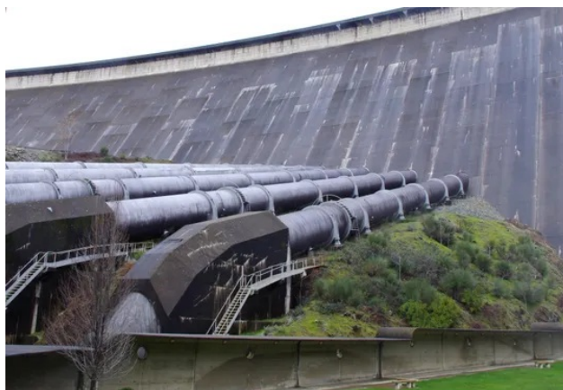
In addition to increasing the amount of water coming down the spillway of Shasta Dam, four of the five turbines were generating electricity Tuesday. (Photo: Damon Arthur/Record Searchlight)
