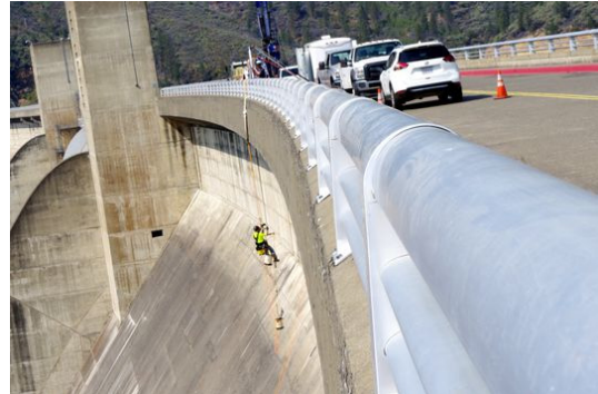
Workers did testing on Shasta Dam in 2018 to determine whether it could withstand having an additional 18 1/2 feet of concrete placed on the crest of the dam. (Photo: Damon Arthur/Record Searchlight)
