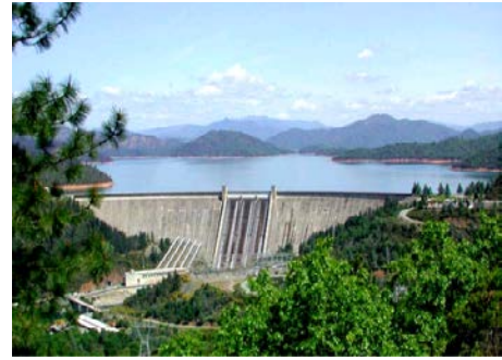
Present Shasta Dam
