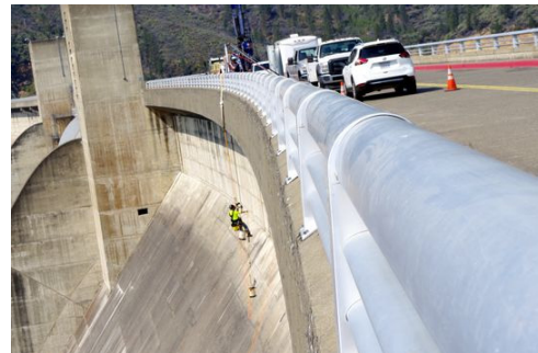
Nathan Morgan hangs over the side of Shasta Dam on Thursday. Morgan and others were drilling holes in the dam to test the strength of the concrete in preparation for raising the height of the dam. (Photo: Damon Arthur/Record Searchlight)
