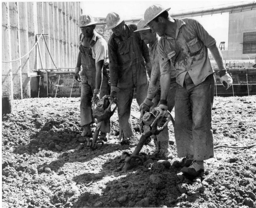
Workers vibrating concrete blocks. (United States Bureau of Reclamation photo)
