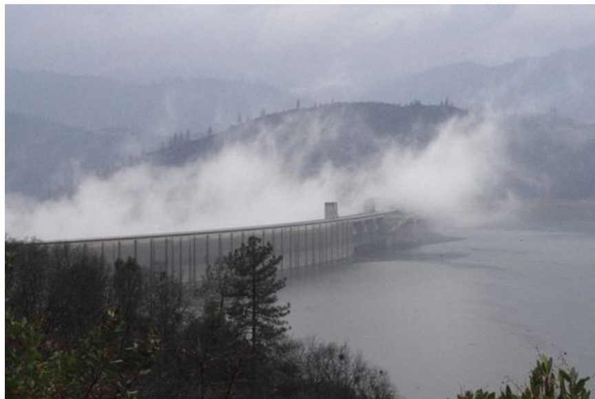
Federal officials want to raise the height of Shasta Dam to store more water in Lake Shasta. (Photo: Damon Arthur/Record Searchlight)
