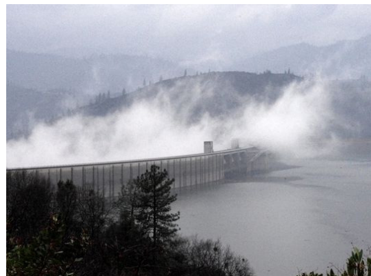
Federal officials want to raise the height of Shasta Dam to store more water in Lake Shasta. (Photo: Damon Arthur/Record Searchlight)
