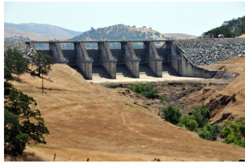
Merced Sun-Star - SUN-STAR PHOTO BY MARCI STENBERG MID wants to raise the Lake McClure spillway facilities by 10 feet with its new Exchequer Spillway Modification Project. It would not be raising the New Exchequer Dam, just the spillway, and the legislation would allow for some occasional short-term increases in the level of Lake McClure not to exceed elevation 877 feet.
