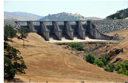
MARCI STENBERG/MERCED SUN-STAR FILE Merced Irrigation District wants to raise the Lake McClure spillway facilities by 10 feet with its new Exchequer Spillway Modification Project. It would not be raising the New Exchequer Dam, just the spillway, and the legislation would allow for some occasional short-term increases in the level of Lake McClure not to exceed elevation 877 feet.
