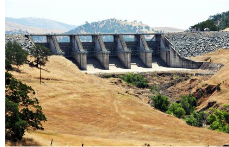
Merced Sun-Star - MARCI STENBERG Merced Irrigation District spillway gate at the main reservoir, Lake McClure a half mile or more away from the dam on the northwest end of the lake.
