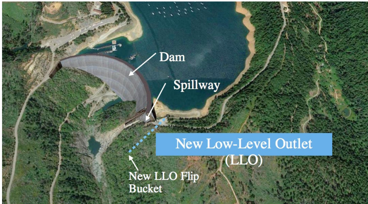
The Yuba County Water Agency proposes to build a new, larger spillway at New Bullards Bar Dam on the North Yuba River. The new spillway would involve tunneling through the mountainside next to the existing spillway. (Photo credit: Image courtesy Yuba County Water Agency)
