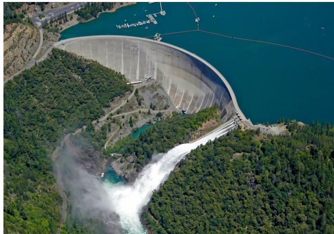
An aerial photo of the Yuba County Water Agency's New Bullards Bar Dam on the North Yuba River in California. A proposed secondary spillway would be built just to the right of the existing spillway at an estimated cost of $160 million.
