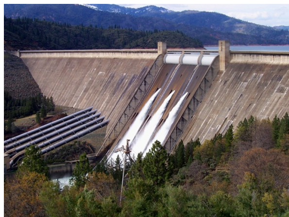
Shasta Dam / US Bureau of Reclamation
