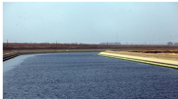
The California Aqueduct brings water from the San Joaquin Delta to Westlands Water District. This photo was taken in 2014 along Avenal Cutoff Road just east of Interstate 5. DANIEL CESAREZ Vida en el Valle/The Fresno Bee
