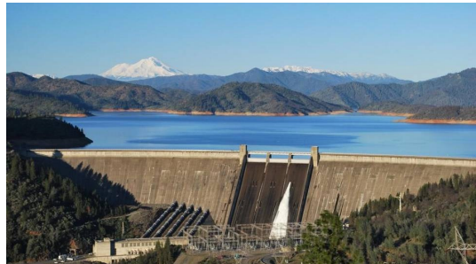
Funds to raise Shasta Dam have already been approved, and Jon Rubin of San Luis and Delta-Mendota Water Authority is supportive of the idea. Contributed
