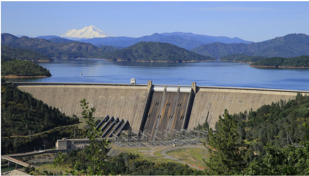
Shasta Dam in Northern California would grow nearly two stories taller under a contentious Trump administration plan. (Allen J. Schaben / Los Angeles Times)
