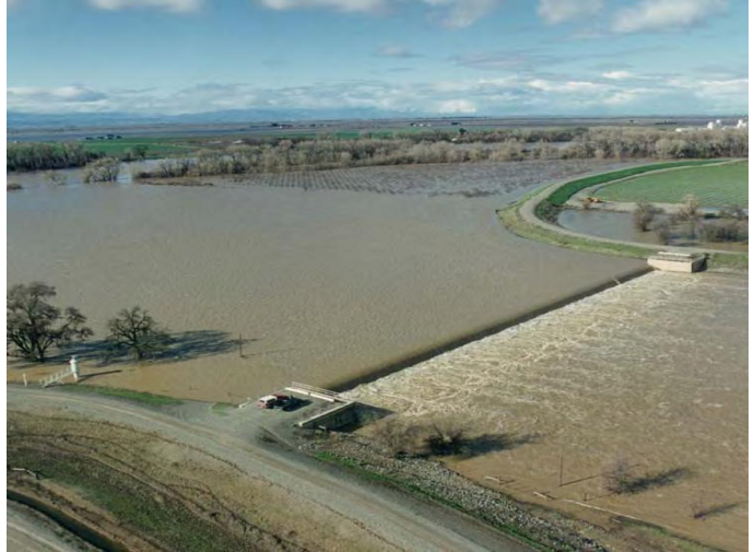
Figure 3, Moulton Weir, January 1997
