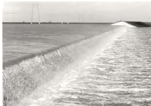
Figure 10, Cache Creek Settling Basin Weir, March 1995
