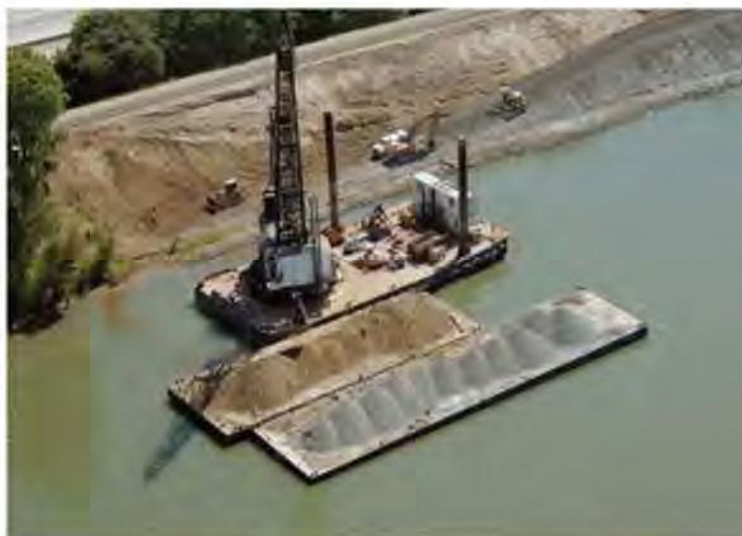
Levee repair site on Sacramento River
