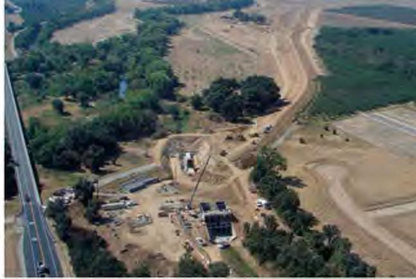
Setback levee being constructed near Bear River
