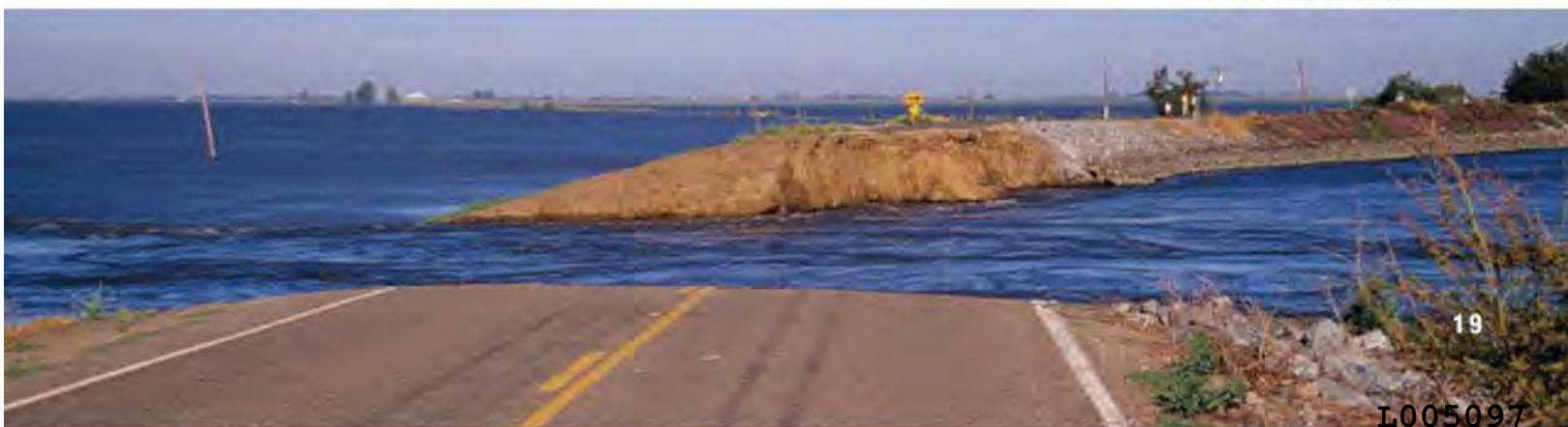
Levee break at Jones Tract
