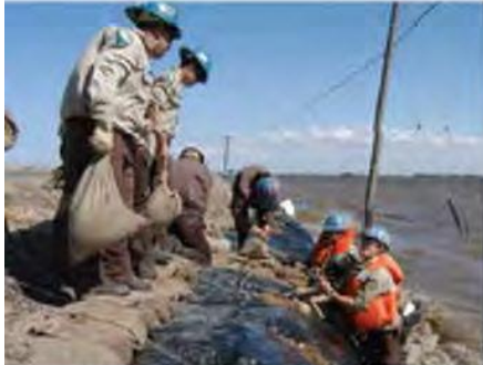
California Conservation Corps workers strengthen a levee during a high water event
