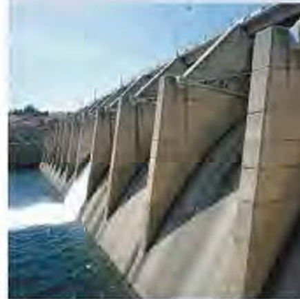
Thermalito Diversion Dam Powerplant
