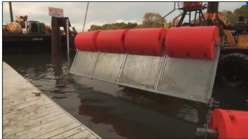
Figure 31. Floating wall being installed near the entrance to Georgiana Slough in 2014 (screen capture from: http://www.youtube.com/watch?v=937bXx9QMn8&feature=youtu.be )
