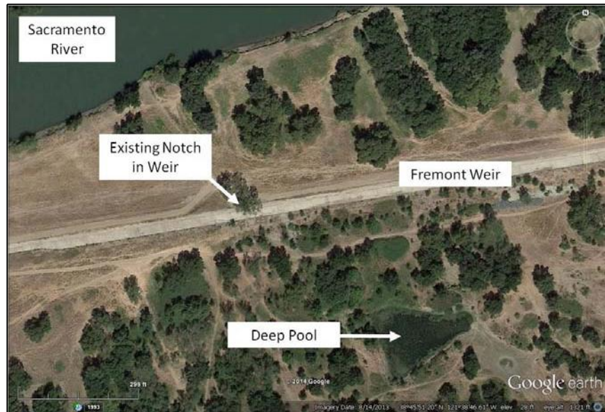
Figure 23. Aerial photograph of the deep pool just downstream of Fremont Weir where adult fish have been stranded.
