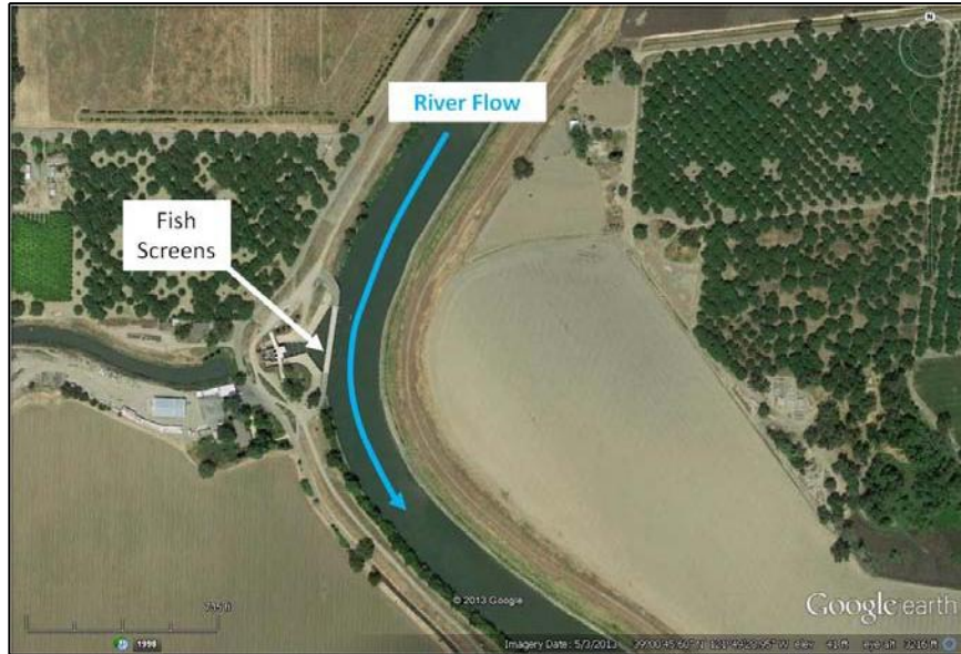
Figure 5. Aerial photograph of an example of an existing Sacramento River flat-plate fish screen located on an outside river bend to maintain high sweeping velocities. Water velocities passing the screen typically range between 2 to 4 feet/second (USBR 2006).
