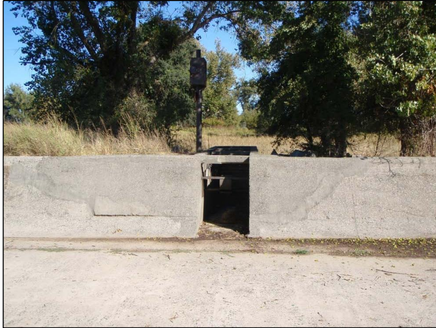
Figure 22. The Fremont Weir “fish ladder”. Photo by Dave Vogel.
