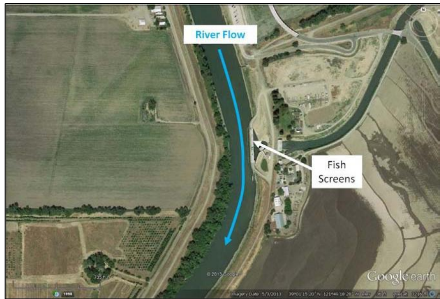
Figure 4. Aerial photograph of an example of an existing Sacramento River flat-plate fish screen located on an outside river bend to maintain high sweeping velocities.
