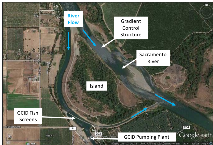
Figure 20. The GCID Hamilton City Pumping Plant and associated features of the Fish Screen Improvement Project.
