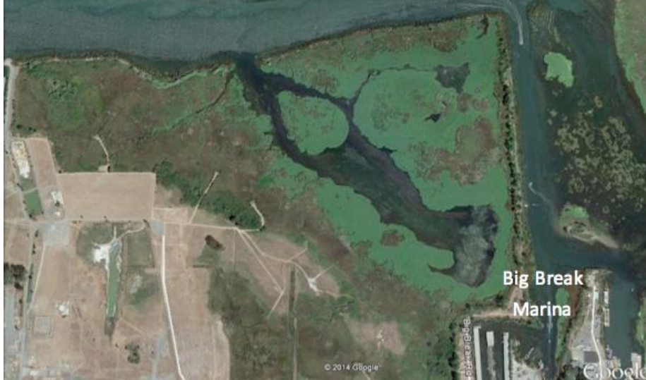
Figure 6. The west end of Big Break is a failed chemical company mitigation site. Some of the chemical waste facilities can be seen at the lower left. The site is virtually abandoned. Big Break Marina is located at the right.
