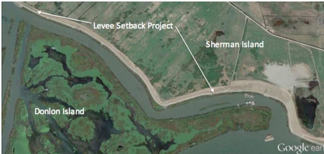
Figure 12. The Sherman Island Levee Setback Project is shown on the southwest shoreline of Sherman Island on Mayberry Slough across from Donlon Island as a narrow strip of green on a new near-white rock levee.
