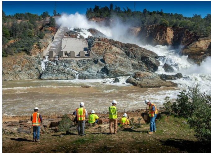
State workers check on the flow of Oroville Dam's battered main spillway in mid-March. A preliminary analysis by the U.S. Army Corps of Engineers cites the presence of substandard materials beneath portions of the spillway, problems with the underlying drainage system and other woes as possible causes of the spillway's fracture. Hector Amezcua hamezcua@sacbee.com
