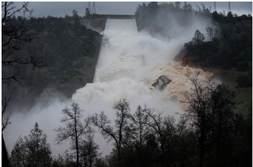
The California Department of Water Resources and host of collaborating agencies continue to monitor the Lake Oroville spillway flows late Thursday afternoon as 35,000 cubic feet per second (cfs) of water was released over the damaged spillway. More erosion is expected, but the releases will help operators absorb the inflow of the storm waters expected Thursday evening and Friday. DWR first noticed erosion on the spillway Tuesday morning and shut off flows to investigate. (Courtesy of the California Department of Water Resources)
