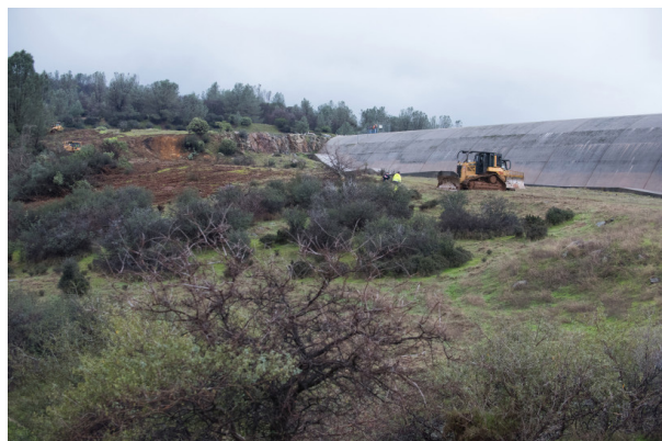
The California Department of Water Resources is preparing a contingency plan for the potential use of the Lake Oroville emergency spillway, as DWR clears trees, rocks and other debris from the hillside near the dam where water would flow. Approximately 50 to 100 acres of trees and brushes could be affected by water releases. The removal would reduce the potential debris flow into the diversion pool and Feather River in Butte County. (Courtesy of the California Department of Water Resources)
