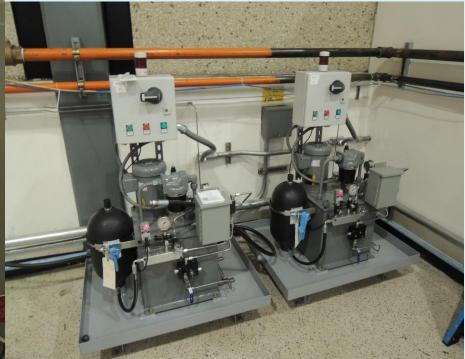
Reinstalled FCVs, 5 days of Validation Testing w/DWR, MWH, and USU in July 2014 which was also witnessed by IOUE and DSOD – RVOS limited to 2000 cfs WO BR
