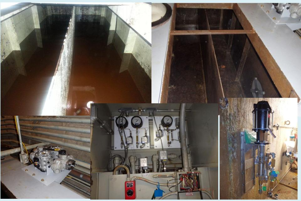
RSV trunion hydraulic system cleaned, and new piping and Duplex filter added. RSV seats converted to water pressure actuation due to past experience with oil/water mixing past seat O-rings. New PRW pressure switches for auto-shut down.
