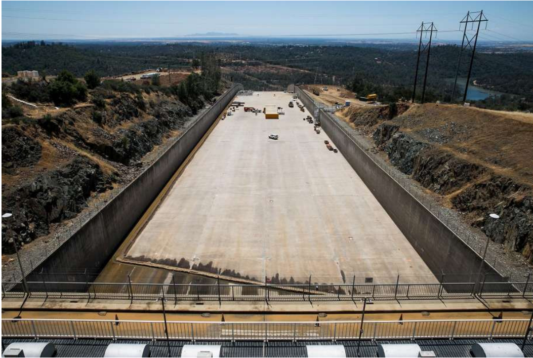
The upper 1,000 feet of the main 3,000-foot-long chute at the Oroville [Dam] is being patched and waterproofed, then rebuilt next summer because there just isn't time to do it this year. Photo: Mason Trinca, Special To The Chronicle
