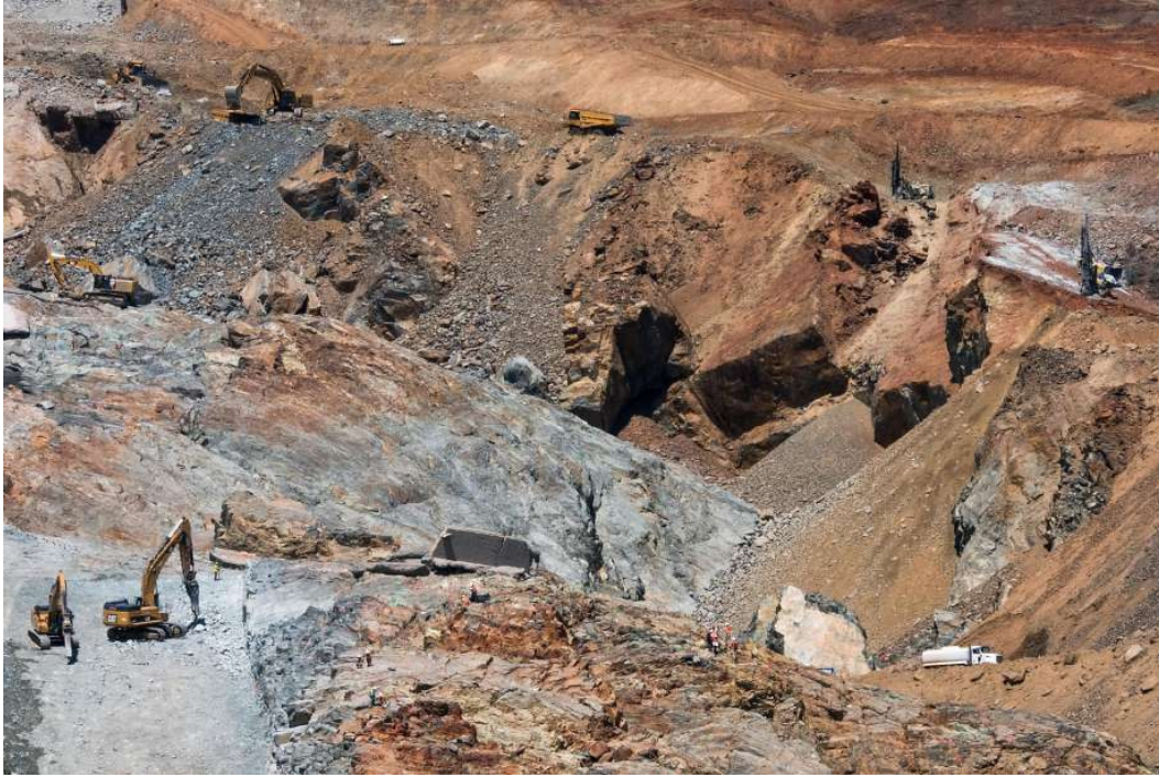
Rebuilding begins at the Oroville Dam after weeks of demolishing 2,000 feet of the compromised main spillway with explosives. Photo: Mason Trinca, Special To The Chronicle
