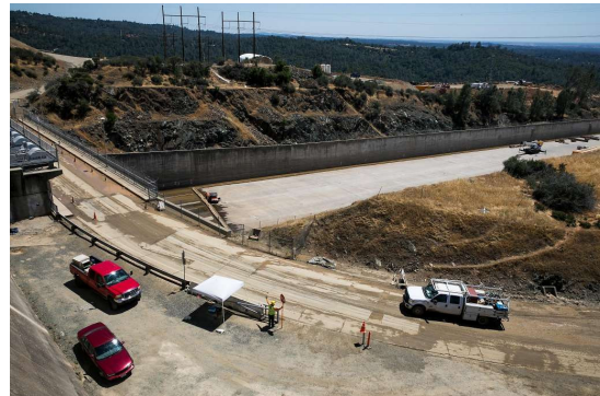
Photo: Mason Trinca, Special To The Chronicle Reconstruction continues on the upper chute of the main spillway at the Oroville Dam, where the workforce is expected to rise from 200 to 500 on the huge project
