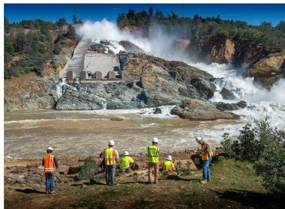
Department of Water Resources workers check on the flow of the Oroville Dam's main spillway on March 17 after water resumed flowing down the fractured main spillway after a three-week shutdown. Hector Amezcua hamezcua@sacbee.com
