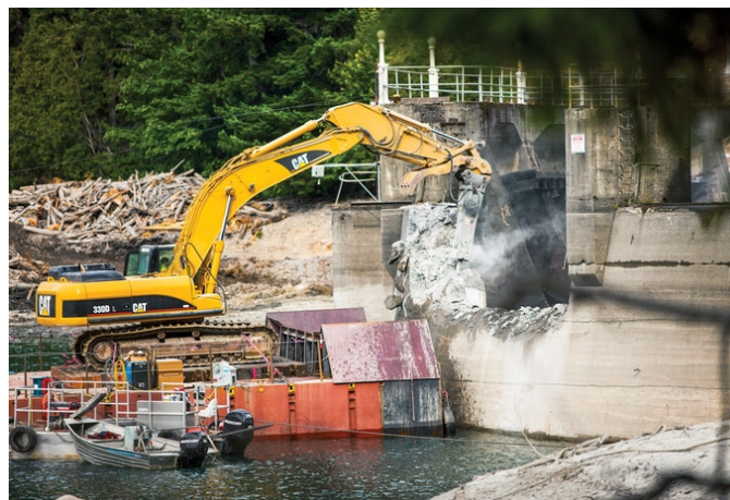
A barge-mounted excavator hammers away at Glines Canyon Dam in Washington, the largest dam removal in U.S. history. Photo/Ben Knight
