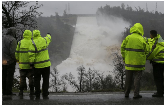
In this Feb. 9, 2017, file photo, water rushes down the damaged Oroville Dam spillway. (AP Photo/Rich Pedroncelli, File)
