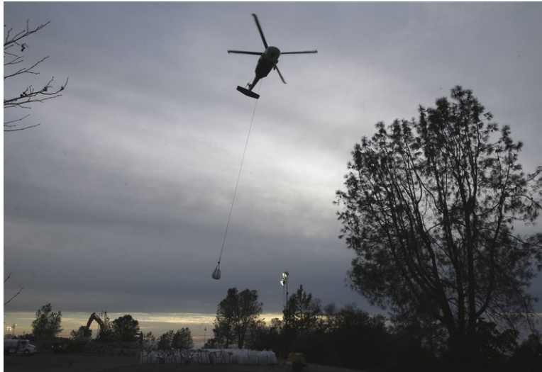
In this Feb. 13, 2017, file photo, a helicopter takes off with a bag filled with rock to be dropped in a hole on the lip of the dam's emergency spillway. (AP Photo/Rich Pedroncelli, File)
