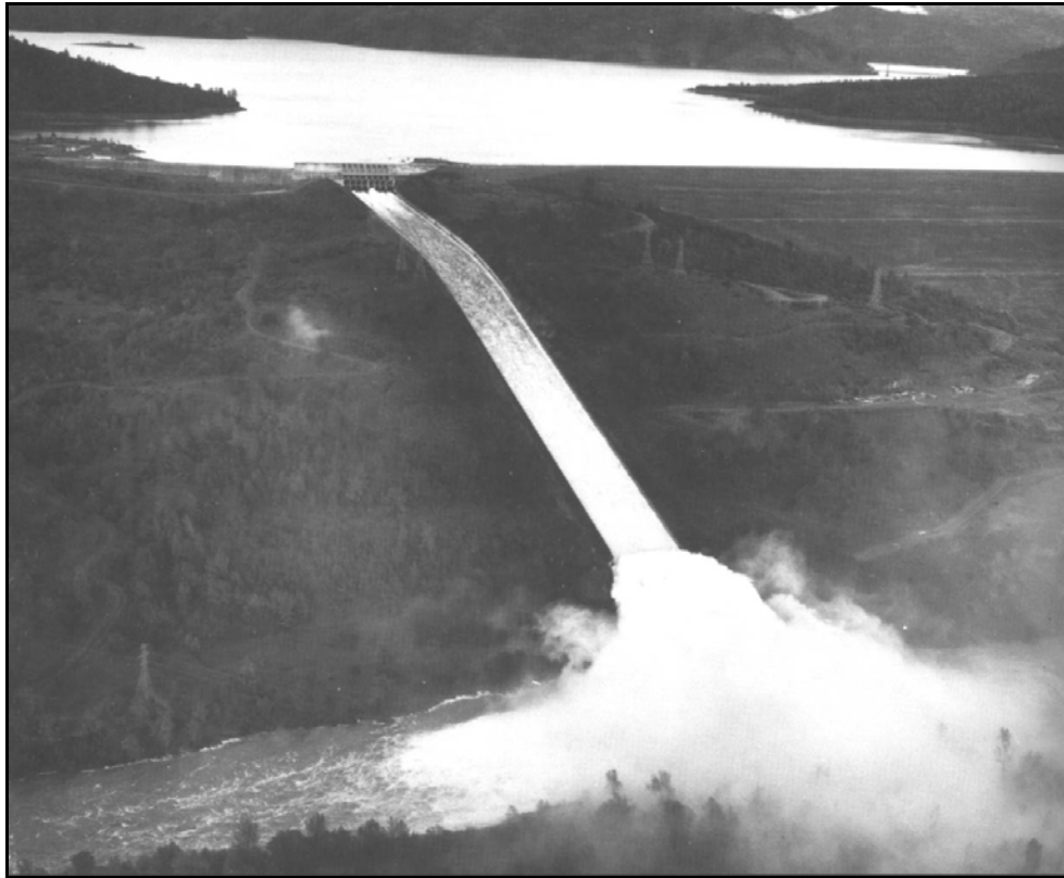
1986 main service spillway operations. Note the ungated spillway to the left, and transmission line towers and road downstream. ACE required design-outflow surcharge operations call for an operational regulated release that could deliver up to this flow over the hillside, reducing and eventually shutting down flows in the service spillway. DWR
