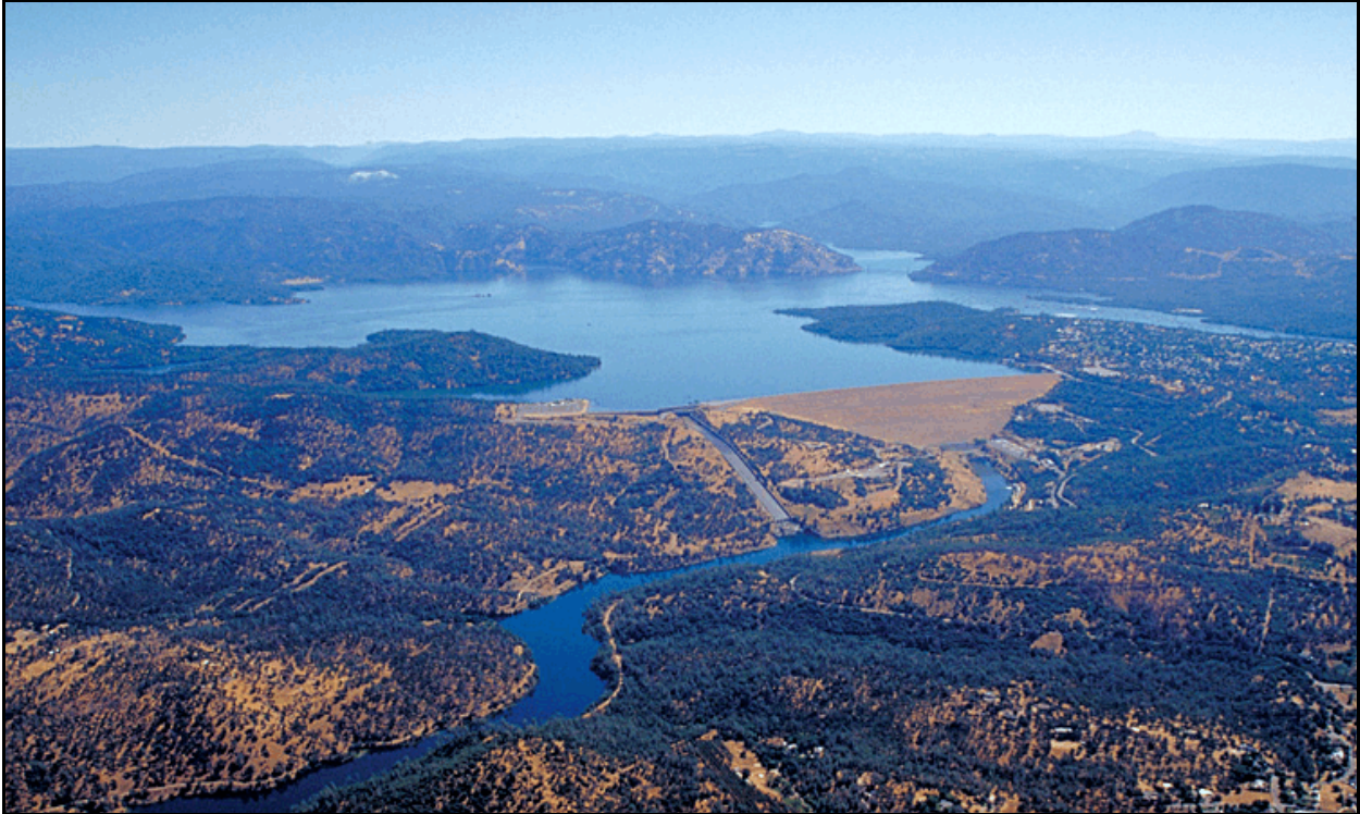
Oroville Dam, Powerhouse, and Spillways. Ungated spillway lip is the lengthy low point to the left of the main service spillway. Regulated design-release out flows of up to 150,000 cfs could flow downslope across the hillside during Corps of Engineers required surcharge operations.
