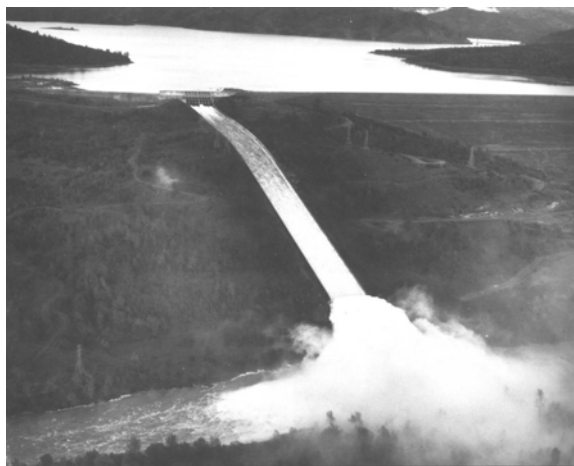
Figure 5. 1986 main service spillway operations. Note the ungated spillway to the left, and transmission line towers and road downstream. ACE required design-outflow surcharge operations call for an operational regulated release that could deliver up to this flow over the hillside, reducing and eventually shutting down flows in the service spillway.
