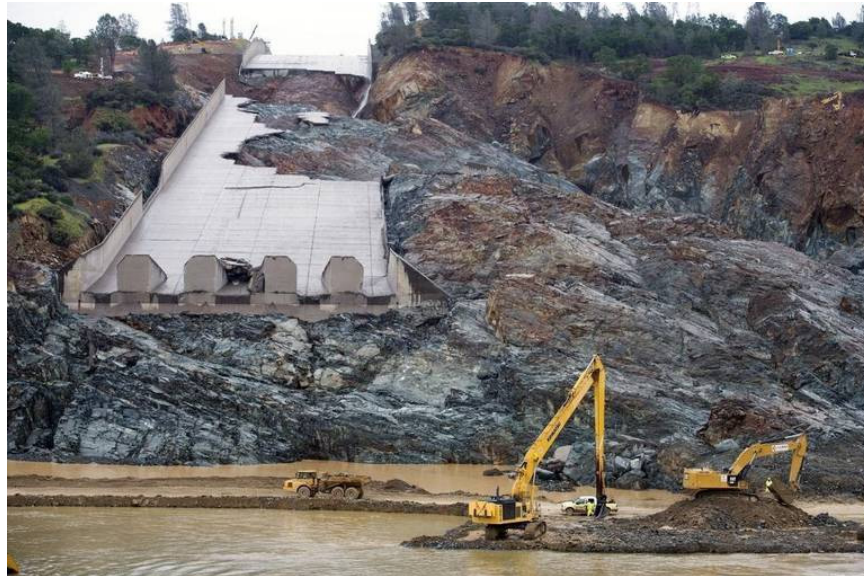
Excavators dredge along the edge of the diversion pool below the spillway at Oroville Dam on April 6 in Oroville, California's top water official said Thursday he's considering releasing redacted copies of safety and progress reports at the troubled Oroville Dam after his office had tried to keep them secret because of terrorism concerns. Randy Pench rpench@sacbee.com
