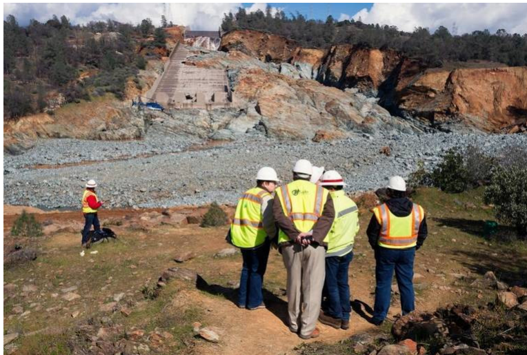
Workers assess damage to Oroville Dam's main spillway in late February. Documents regarding the the spillway's fracture and repair, as well as Gov. Jerry Brown's response to the crisis, have been kept from public view. Paul Kitagaki Jr. pkitagaki@sacbee.com
